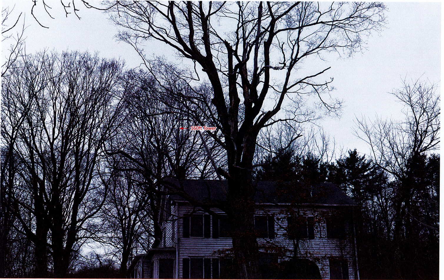
Photo 01 - Airport Road SIMULATED CONDITION
