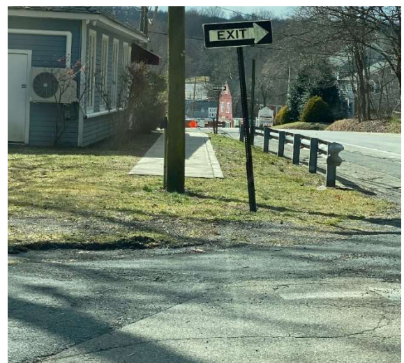
Figure 9 – Sidewalk Dead End
